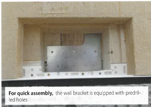
After assembly, the lower portion of the wall bracket and the upper portion of the floor bracket overlap
