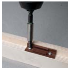
Mount with screws or nails
