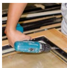
Screw or nail the FIXclip-profile in place
