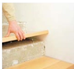
Transfer bore holes
