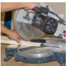
Cut to size glazing bead and FIXclip-profile
