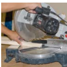
Cut to size glazing bead and FIXclip-profile
