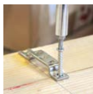
Mount KOMBI bracket with screws
