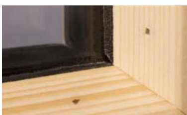
Conventionally fixed glazing bead with visible nails.
