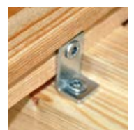
Z-DECK is completely mounted
