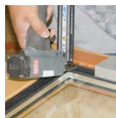
Screw or nail the FIXclip-profile in place
