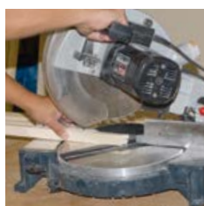
Cut to size glazing bead and FIXclip-profile
